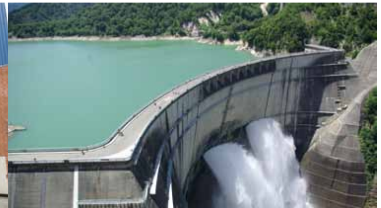
Turbine and pump technology
